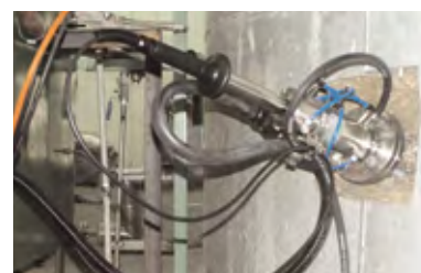
Fig. 2: InTrac 777 e with flushing chamber for automatic cleaning of the pH electrode InPro 3250 SG.
