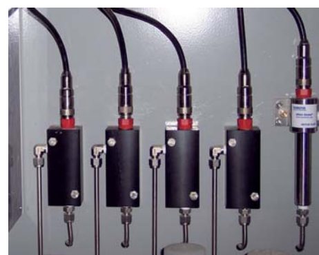
Dissolved oxygen and pH sensors for critical cycle chemistry sample points.
