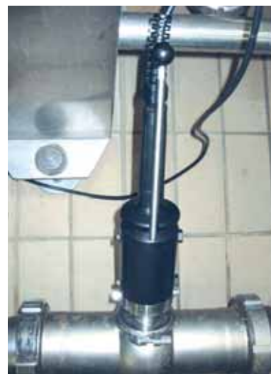
Fig. 1 Retractable housing InTrac 777 mounted in a Tuchenhagen Varivent® housing.
